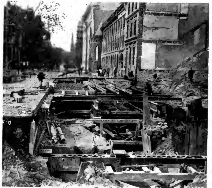
Fig. 4—Viaduct carrying Dorchester street over tracks during erection.
